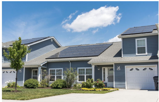
Rooftop solar panels at the Dover Family Housing Community. Credit: Roland Balik via United States Air Force, CC BY 1.0.
