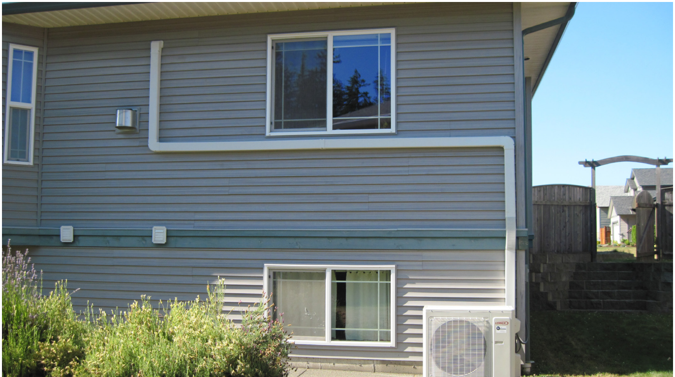
A home with an electric heat pump, which efficiently provides both heating and cooling. Electric appliances such as this, as well as energy efficient design, home batteries and electric vehicles, allow solar panels to meet more of homes' energy needs. Credit: Lani Hudelson via Flickr, CC BY-ND 2.0.
